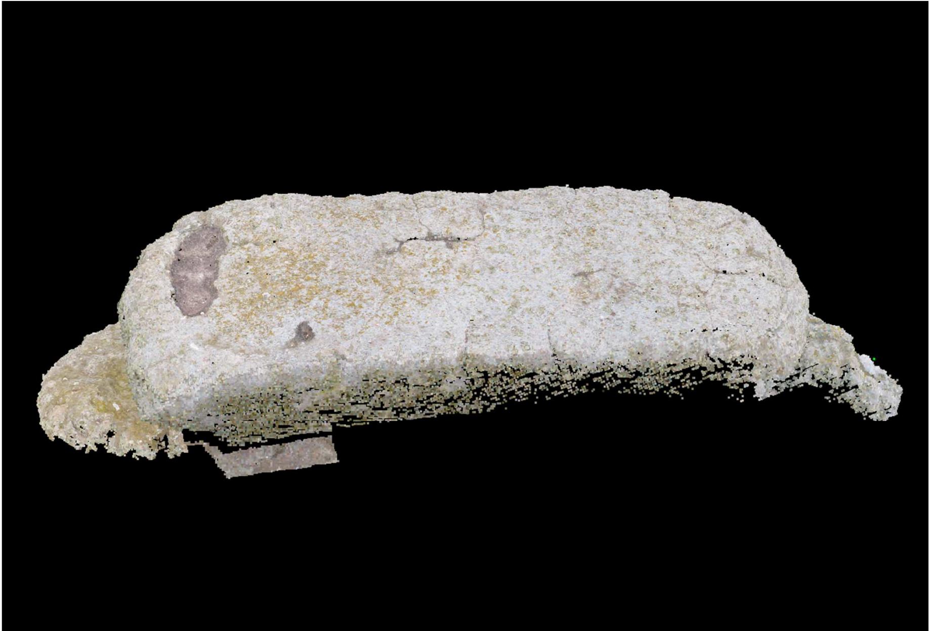
An example of the 1mm resolution, colourised point data available from the resultant digital photogrammetry process, for the upper Stone Lintel No 105.
