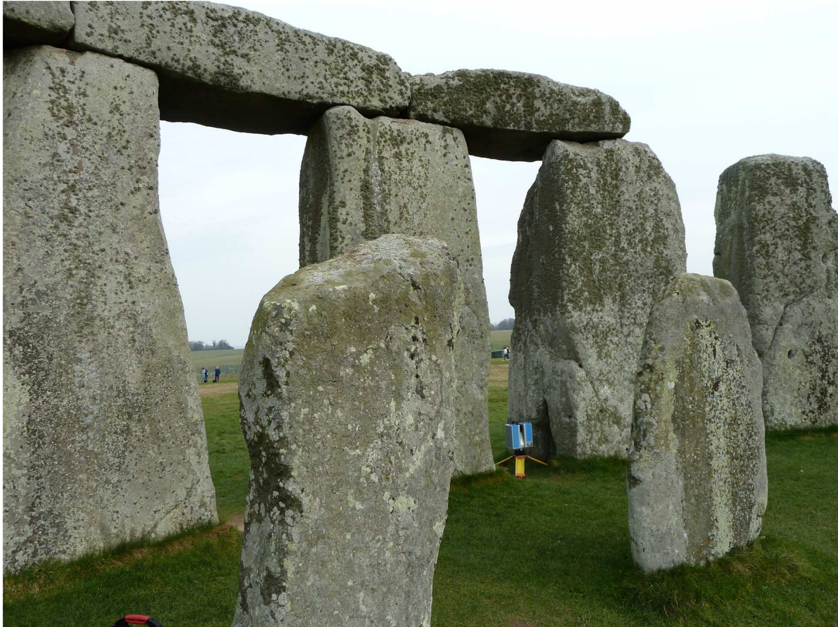
Example of low level laser scan coverage using a reduced height tripod.
