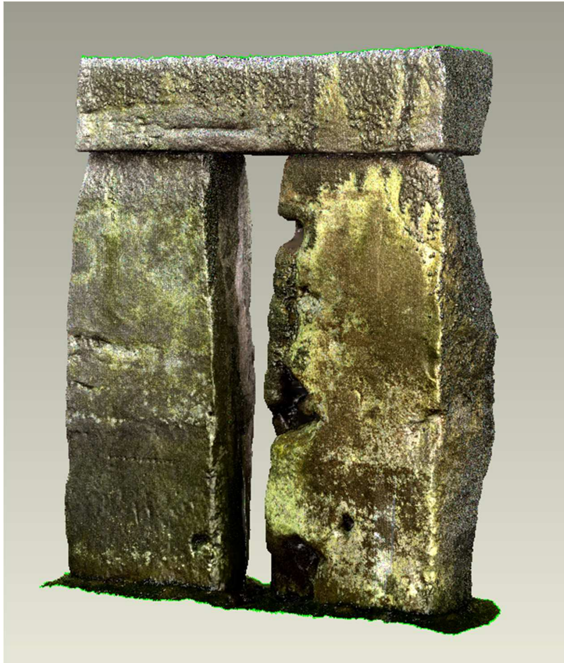
Example of a meshed model surface to stones 53 & 54, with coloured point cloud data overlay.
